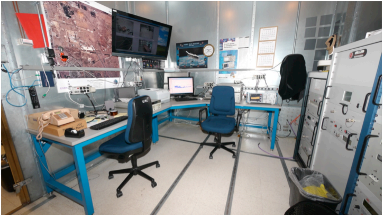
Large EMC Control Console
